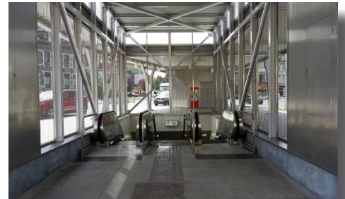
Escalator – Place Albert 1er
